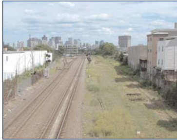
A portion of the proposed right-of-way for the MBTA Green Line extension to Somerville and Medford
