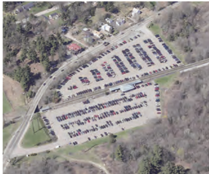
Forge Park/Route I-495 park-and-ride facility in Franklin
